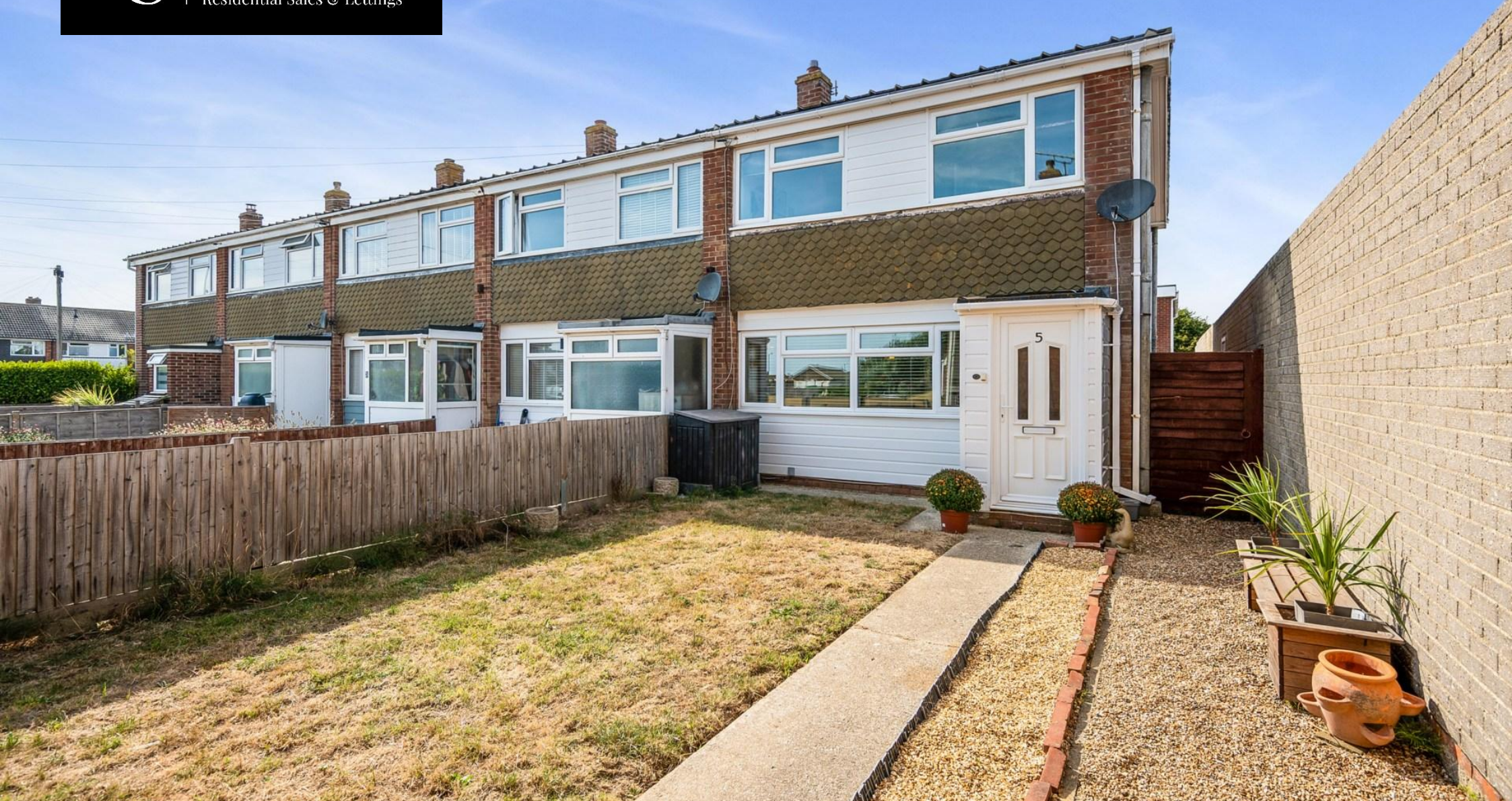
5 Downview Close, East Wittering, PO20 8NS
