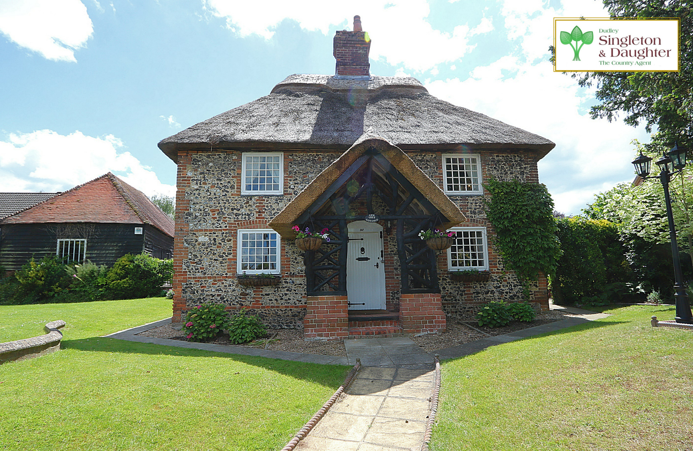
Yew Tree Cottage • Purley Rise • Purley-on-Thames
