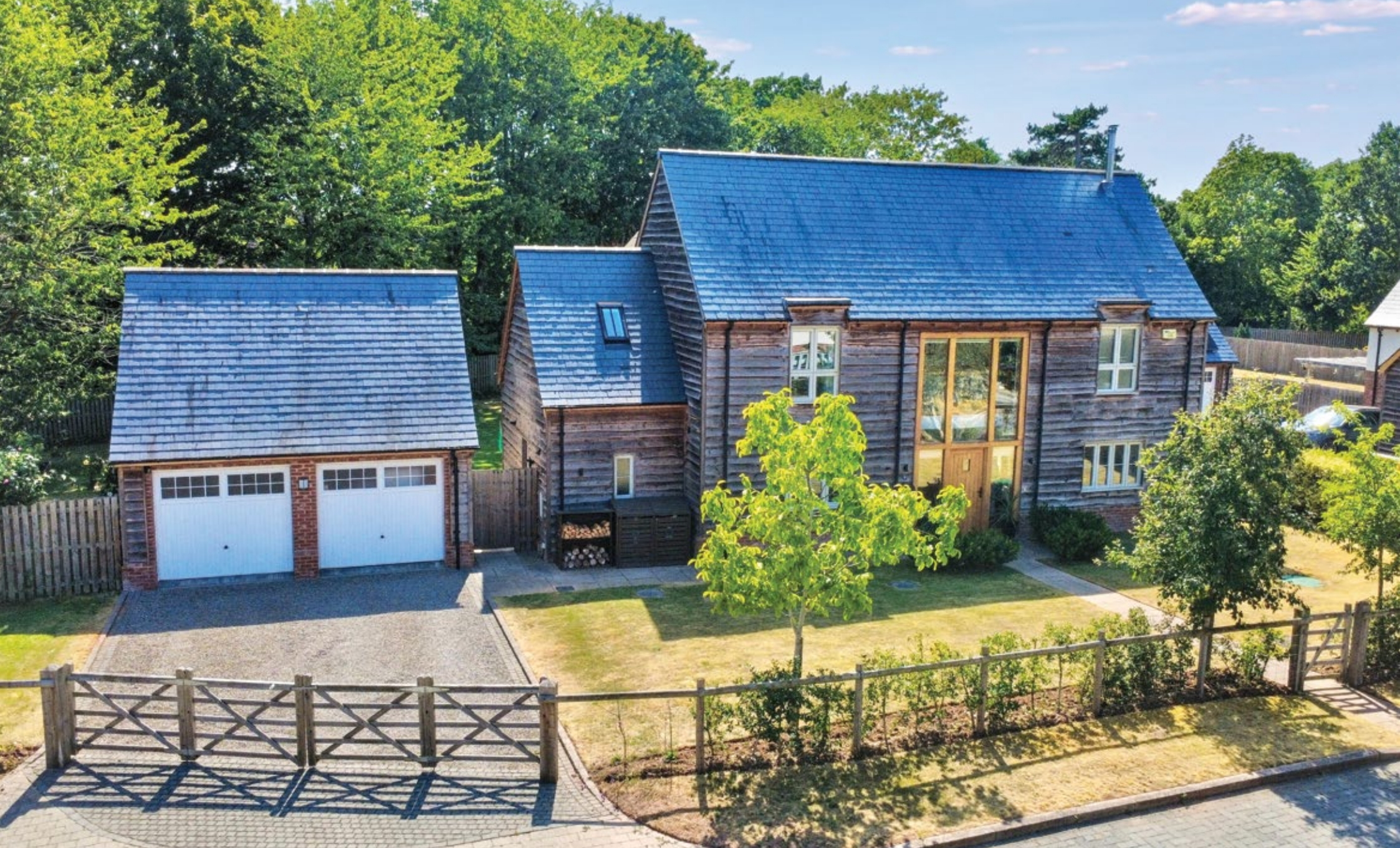
RICHMOND BARN 6 Covent Garden | Redmarley | Gloucestershire | GL19 3LH
