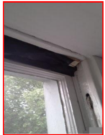
Bedroom 3 Window Window frame/sill - tape repaired
