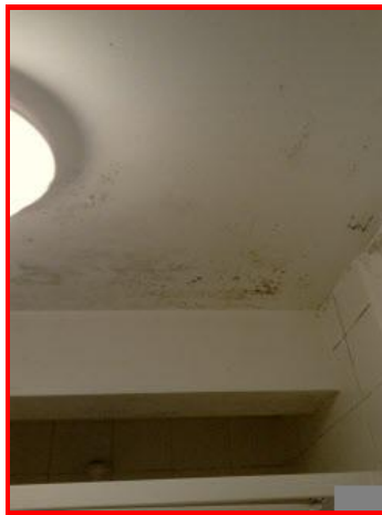
Ceiling finish - black spot mould (heavily)
