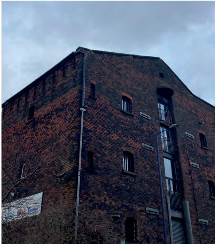
ABOVE: The Grade II listed Mill
