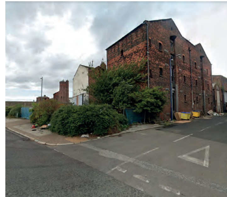
ABOVE - View looking from Blackstone Street
